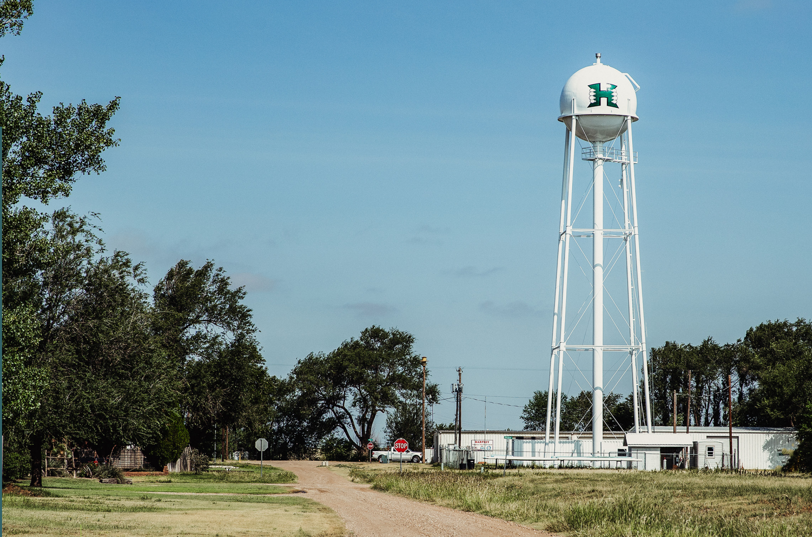
Hartley County Elevated Storage Tank Painting and Rehabilitation COMPLETED IN 2020
